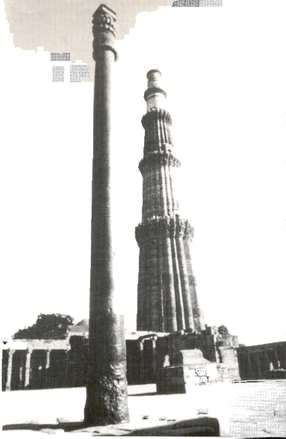
*The Iron Pillar of Delhi — twenty-three feet high — consists of a single piece of iron and is tribute to the metallurgical skill of ancient India. It was constructed in the third or fourth century A.D. and has shown no signs of rusting. In the background is the Qutab Minar, a victory tower, 238 feet high, built more than seven hundred years ago.*
