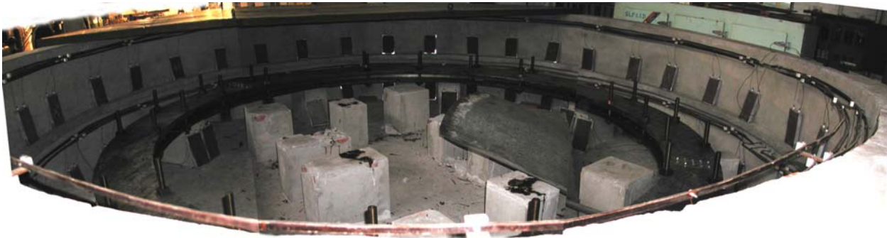
Oven for curing coils
