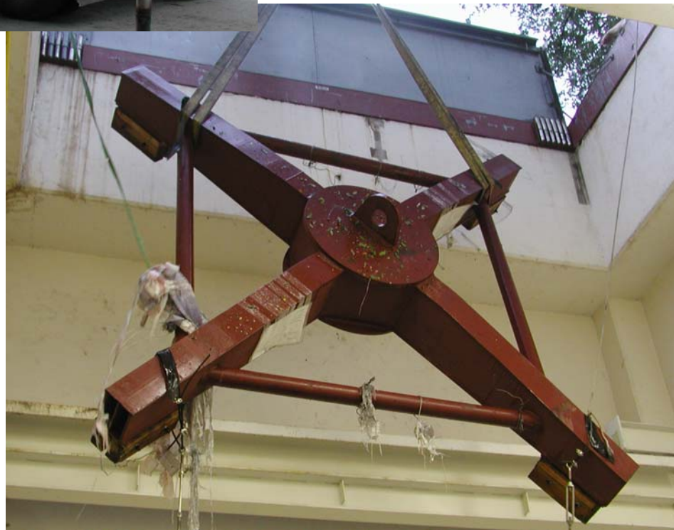
The lifting jig being lowered through the roof hatch into the underground laboratory
